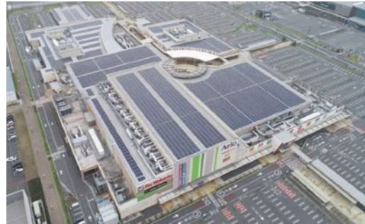
Rooftop solar panels (Ario Ichihara store)
