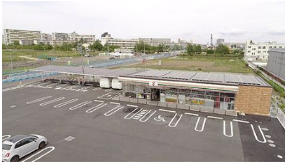
Test store for saving, generating. And storing energy (7-Eleven Misato Hikonari 2-chome store)
