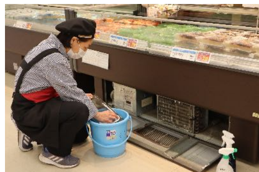
Cleaning the filters on a refrigerator case (York Mart)
