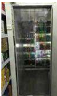
A curtain installed in a walk-in refrigerator
