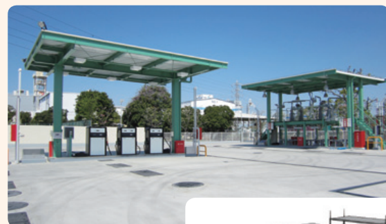
Fuel Storage Station: Above-ground section
