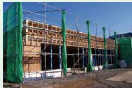
Wooden store under construction
