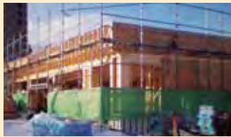
Wooden store under construction
