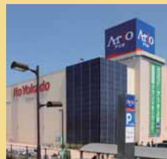
Solar panels installed at the store
