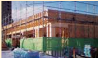
Wooden store under construction
