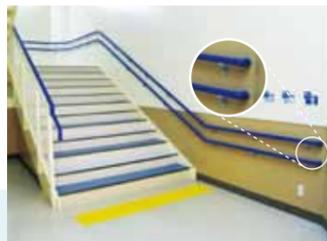
The color is changed at each location with different step levels to make the difference clear. Also, the edge of the handrails is curved toward the wall side to prevent clothing and bags from getting caught.
