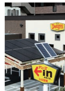
Rooftop solar panels
