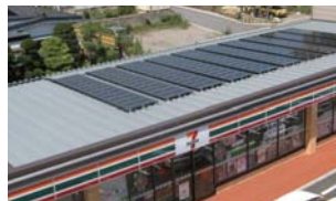
A store with solar panels
