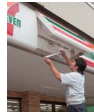
Annual replacement and recycling of fluorescent lights
