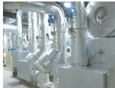
Ice thermal storage system
