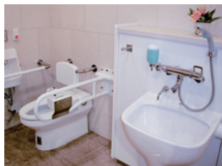
A multi-function restroom with UD consideration (Sogo Shinsaibashi Store)
