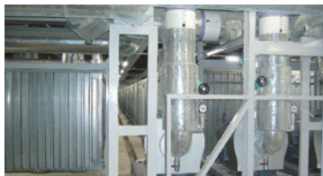
Ice thermal storage system using nocturnal ice-making
