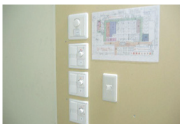
Continuously adjusting lighting facilities fine-tuning light levels
