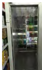
A curtain installed in a walk-in refrigerator
