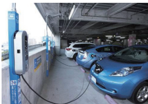
Electric Vehicle Charger
