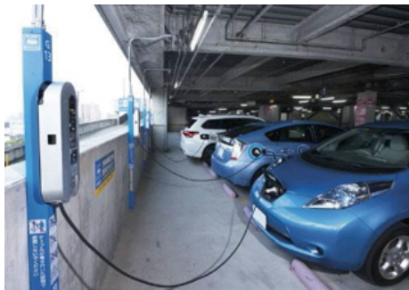
Electric vehicle charger
