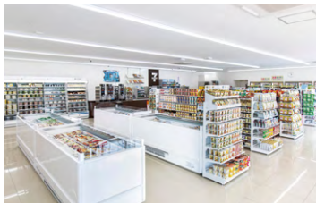
Installation of LED lighting and other energy-saving equipment
