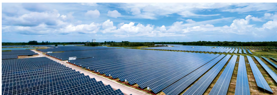
Large-scale solar power facility in Florida
