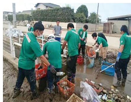
Restoration of a store inundated by the heavy rain of July 2018
