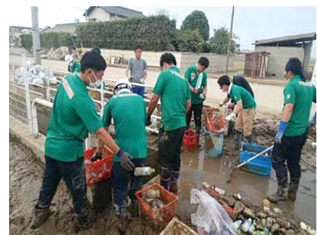
Restoration of a store inundated by the heavy rain event of July 2018
