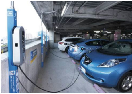
Electric vehicle charger
