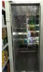
A curtain installed in a walk-in refrigerator
