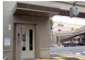
Elevator at a pedestrian overpass
