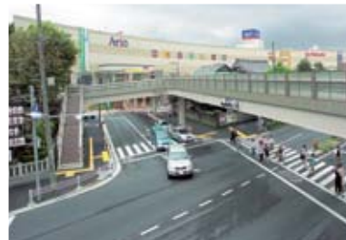
Pedestrian overpasses for avoiding vehicular traffic
