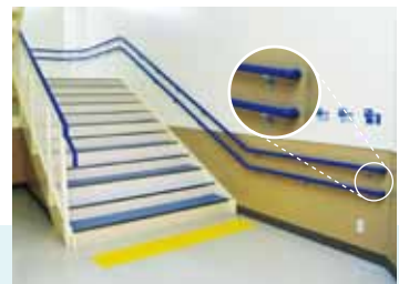
The color is changed at each location with different step levels to make the difference clear. Also, the edge of the handrails is curved toward the wall side to prevent clothing and bags from getting caught.
