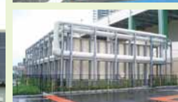
Ice thermal storage system to make ice using electricity during the night while the shopping center is closed, and then utilize the ice for air conditioning during hours of operation.
