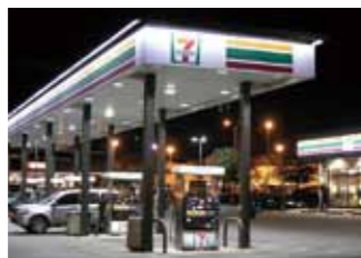
Exterior gas canopy with LED lighting
