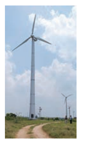
Wind power station in Tamil Nadu State
