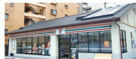
An eco-friendly store equipped with top lights and solar panels
