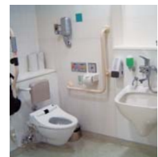
Multi-use restrooms feature wider spaces, and the toilet seat position and washstand height ensure improved accessibility. Audio guidance is also available.
