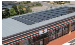
A store with solar panels
