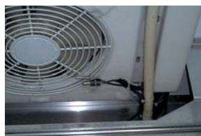
Maintaining the container’s internal temperature with a sensor attached to the cooling fan
