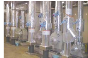
Ice thermal storage system
