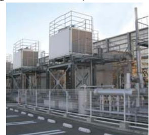
Small cogeneration water-heating system
