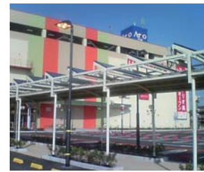
Solar panels in the parking lot
