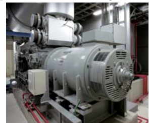
Replacing with new electric generators
