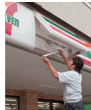
Annual replacement and recycling of fluorescent lights
