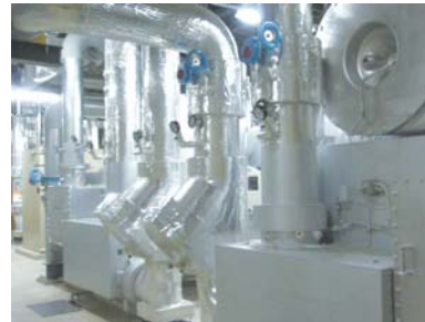
Ice thermal storage system
