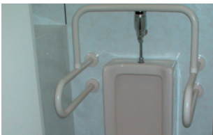
Toilet with handrails installed
