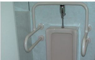
Toilet with handrails installed
