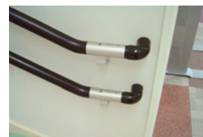
Handrails at two height levels
