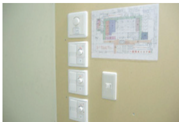
Continuously adjusting lighting facilities fine-tuning light levels
