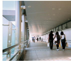
Pedestrian overpass connecting the station and our store
