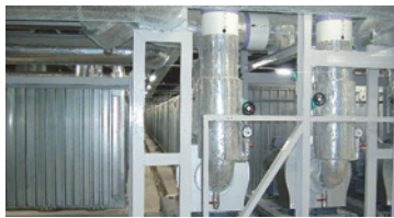
Ice thermal storage system using nocturnal ice-making
