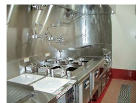
Electricity-powered kitchen equipment with less energy use and CO 2 emissions
